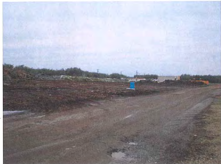
FIGURE 1 GENERALLY SOUTH-EAST VIEW OF TRANSFER STATION INTERIOR
