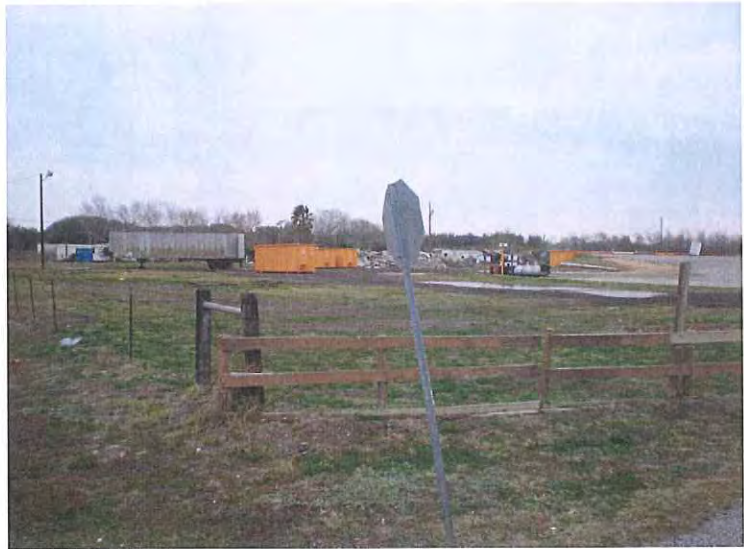
FIGURE 11 SOUTHWEST TRANSFER STATION PERIMETER FENCE
